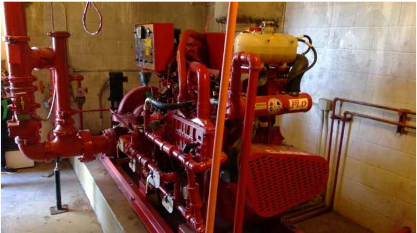
Fire Pump - Diesel
