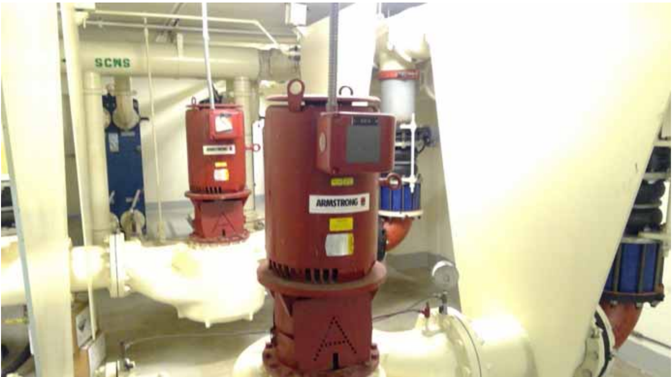
Cooling Tower Pumps
