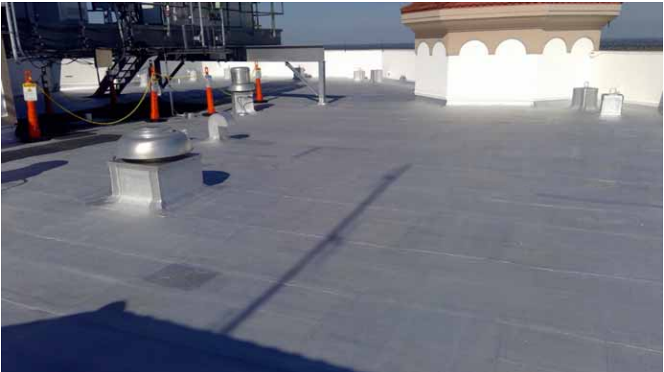
Tower Roof - Modified Bitumen
