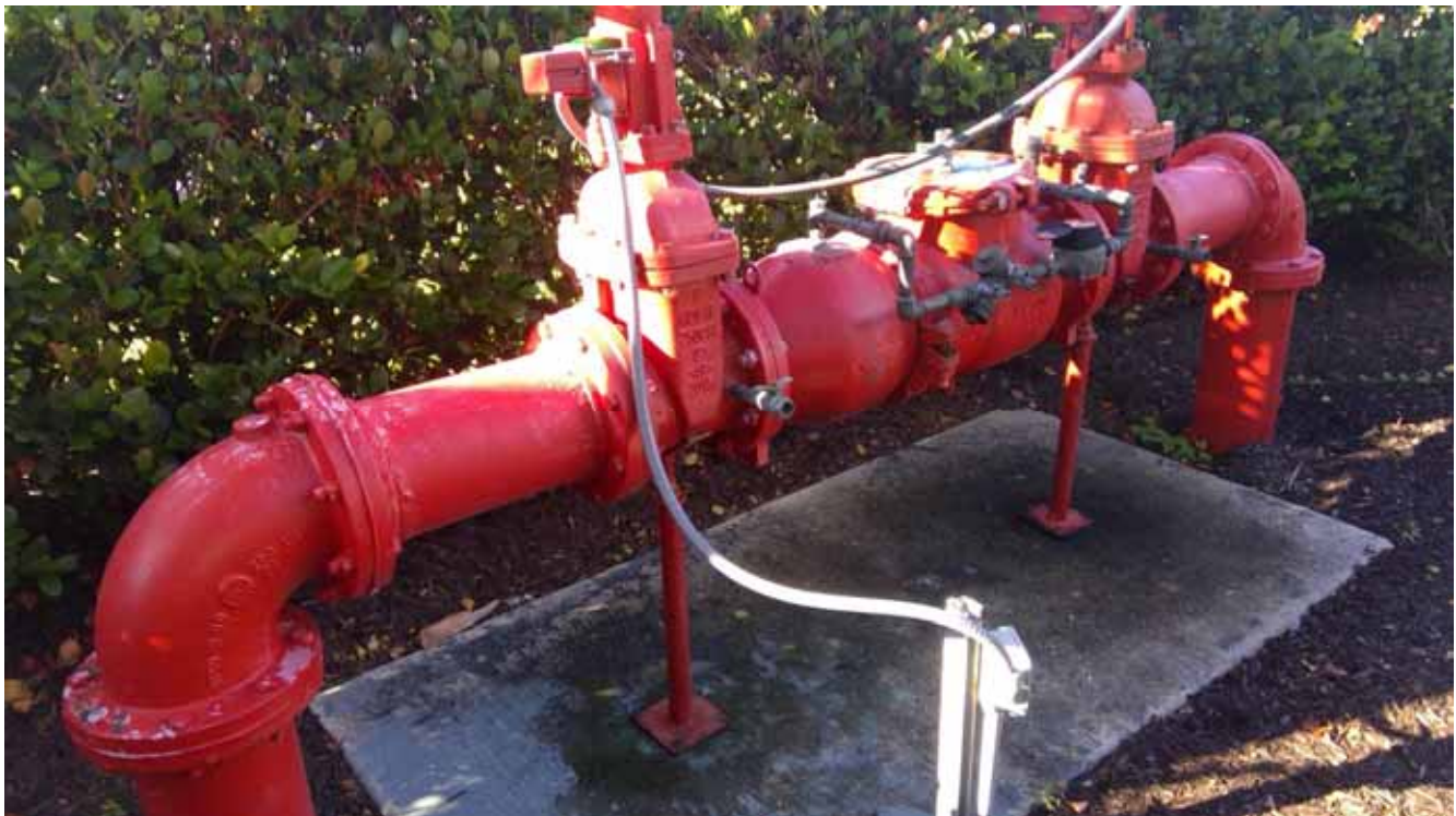
Backflow Preventer - Sprinklers
